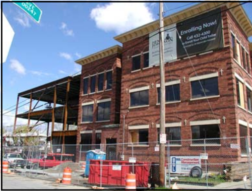
In early May, the side addition is framed and the cement blocks are being put in place, above and at right .
