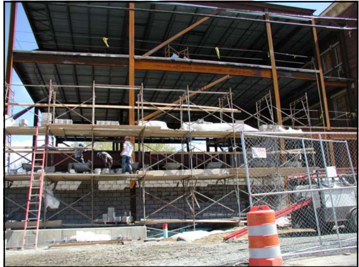
In early May, the side addition is framed and the cement blocks are being put in place, above and at right .
